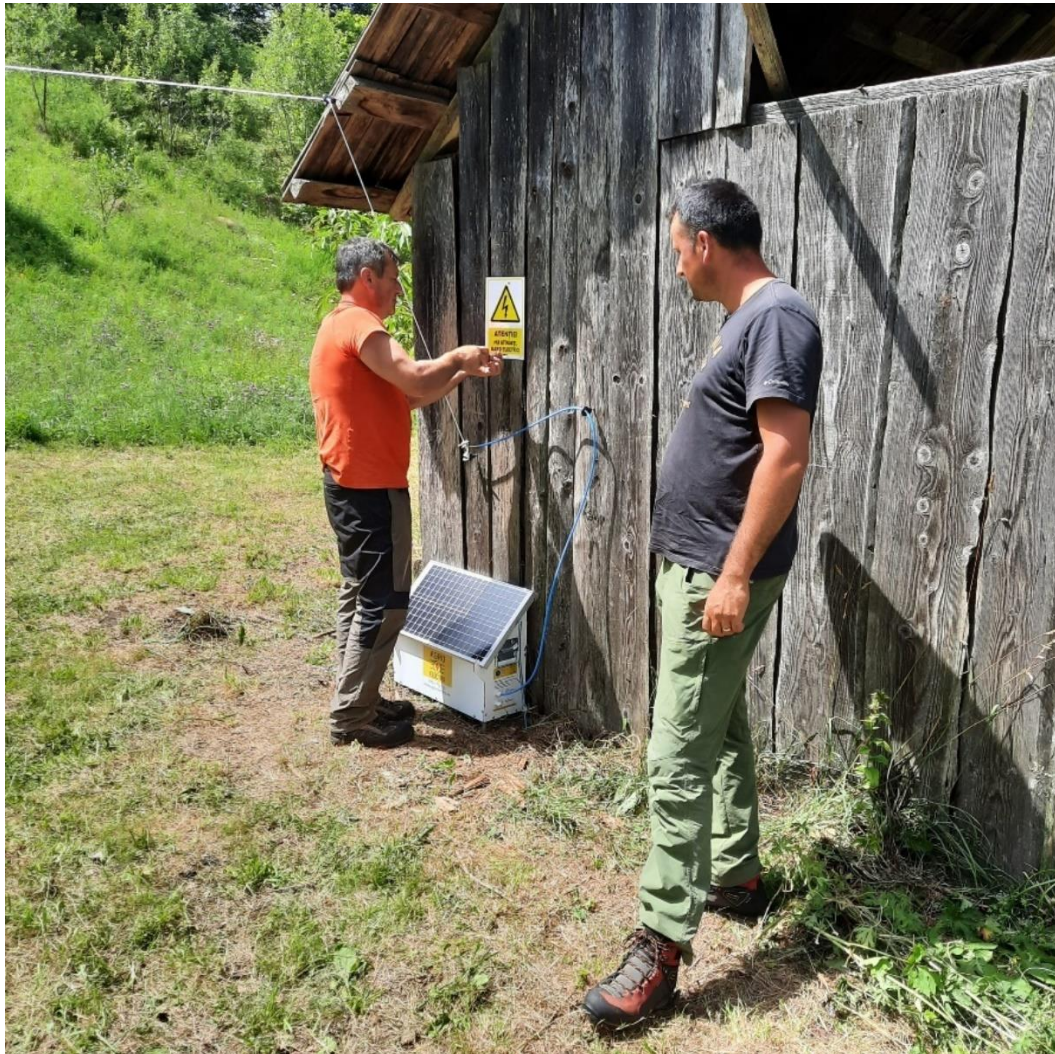
Imagine 47-49 Montare gard electric
